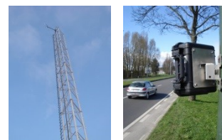
Figure 9 - Automatic anemometer and weather vane at the meteorological mast.
